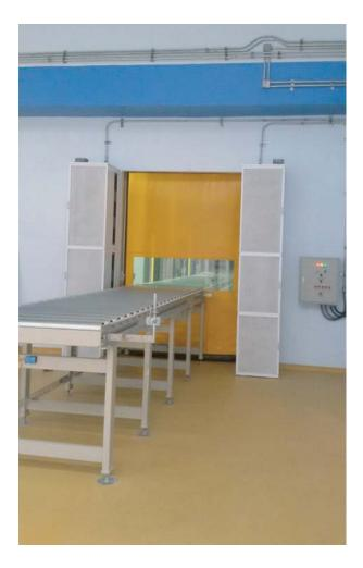
X-Per VQ-9 series of vertical Air Partition are designed specially for insect blocking application in industrial environment. Capable of delivering a maximum airflow velocity of 24 m/s and a maximum airflow volume of 18,000 CMH.
